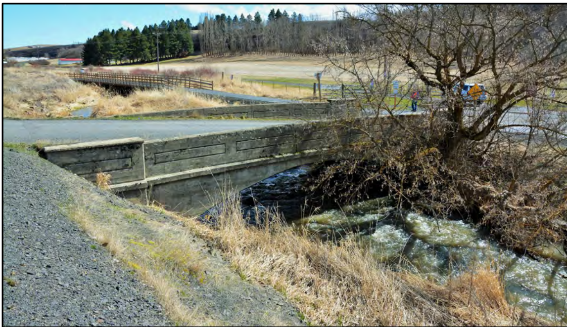
Figure A-78. Wood Bridge (Field Number WCLB-11), west side; view to the southeast (photograph courtesy of Whitman County Public Works).
