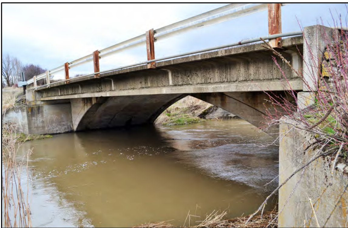
Figure A-10. McLeod Bridge (Field Number WCLB-2), east side – note girder added to widen bridge; view to the south.
