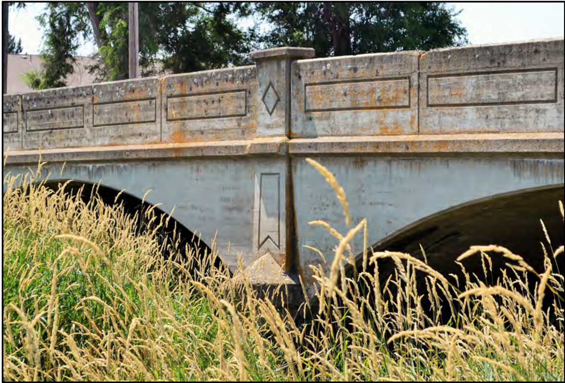
Figure A-45. Colton Bridge No. 37 (Field Number WCLB-7), detail of east side and central pier; view to the southwest.
