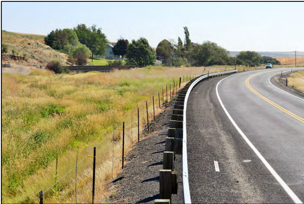
Figure A-102. Rhodes Bridge (Field Number WCLB-15), west side, left, State Route 23, right; view to the northeast.
