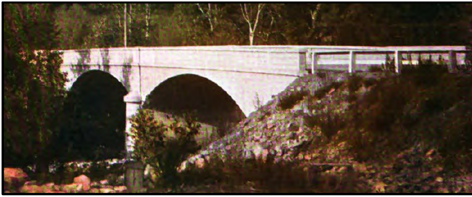
Figure 14. Two-span Peshastin Creek Bridge, Leavenworth, Washington, built 1920 (Luten 1924:33)
