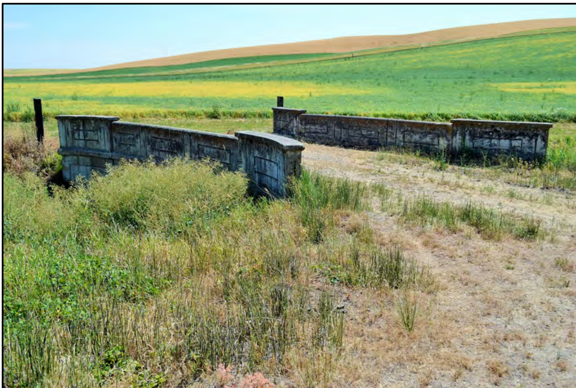
Figure A-98. Bridge No. 318 (Field Number WCLB-14), north approach and east side; view to the southwest. Note curvature of abutments and abutment parapets.
