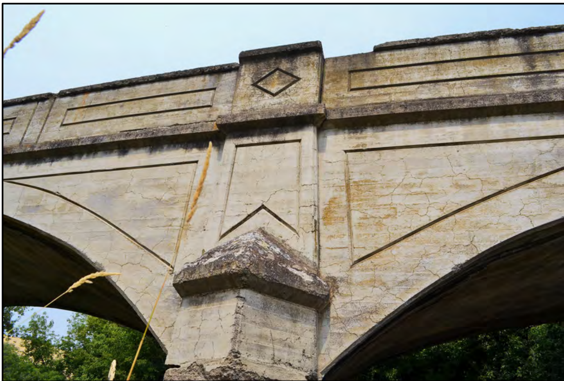
Figure A-119. Sanders Bridge (Field Number WCLB-17), detail of central pier on south side; view to the northwest.
