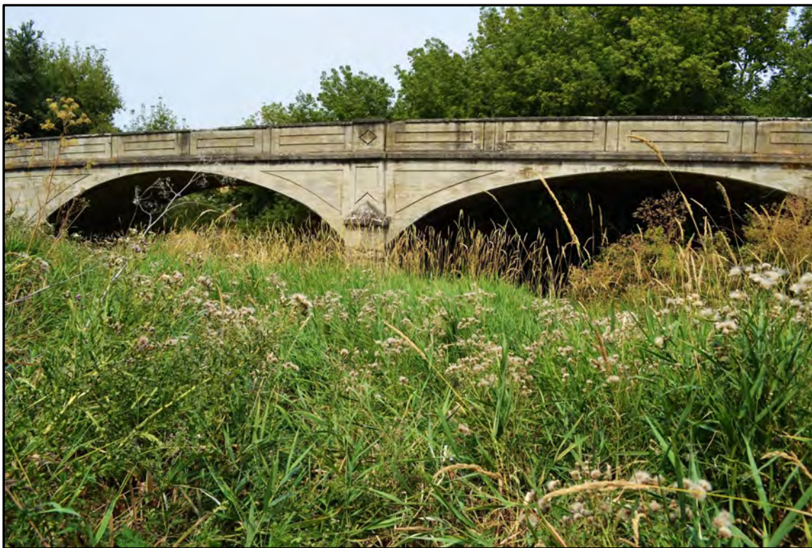
Figure A-117. Sanders Bridge (Field Number WCLB-17), south side; view to the northwest.
