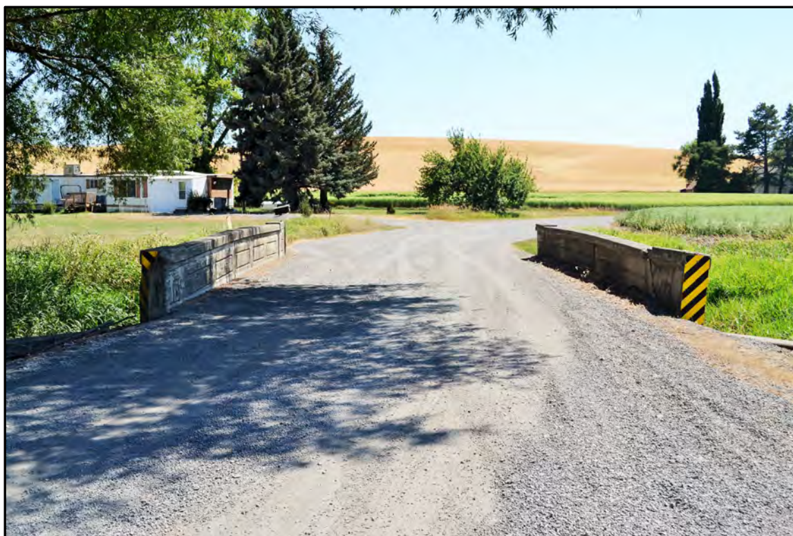
Figure A-31. Staley Bridge (Field Number WCLB-5), north approach; view to the south.
