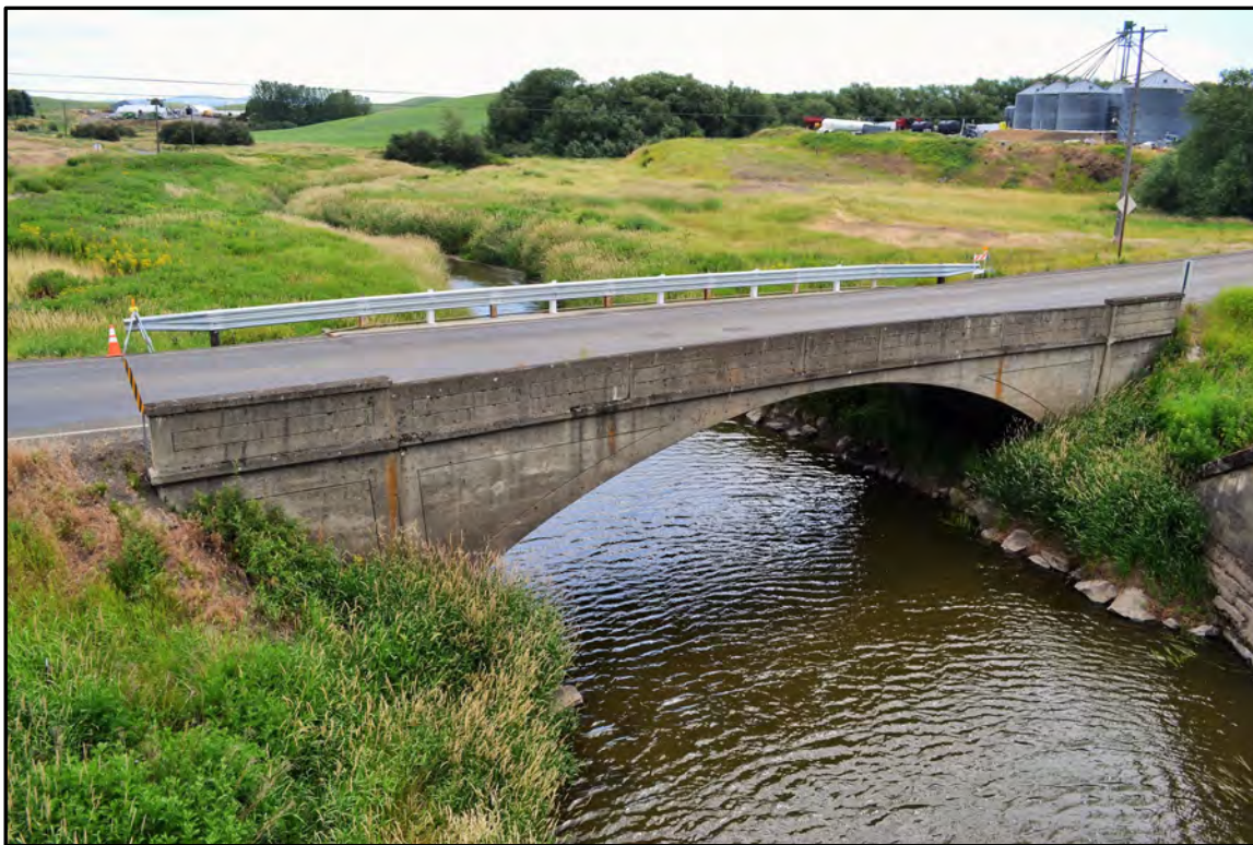
Figure A-9. McLeod Bridge (Field Number WCLB-2), west side; view to the east.
