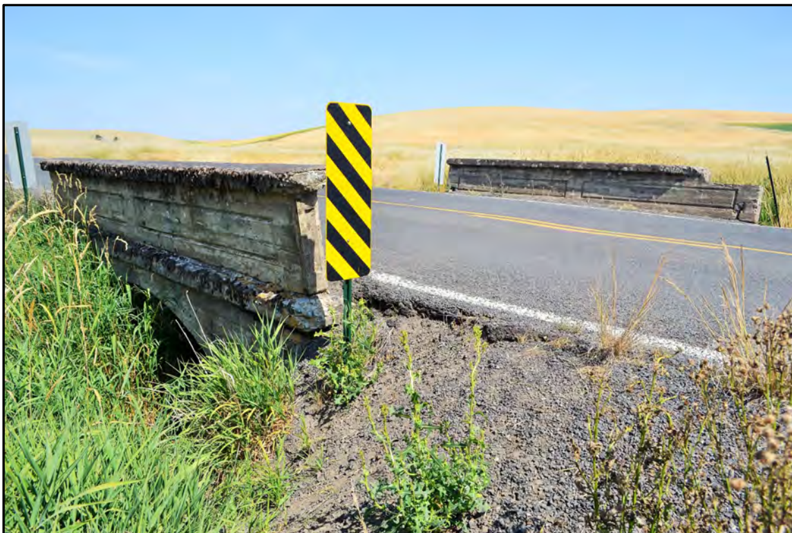
Figure A-39. Colton Bridge (Field Number WCLB-6), west side; view to the east.
