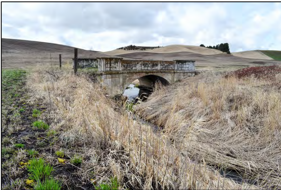
Figure A-96. Bridge No. 318 (Field Number WCLB-14), east side; view to the west.
