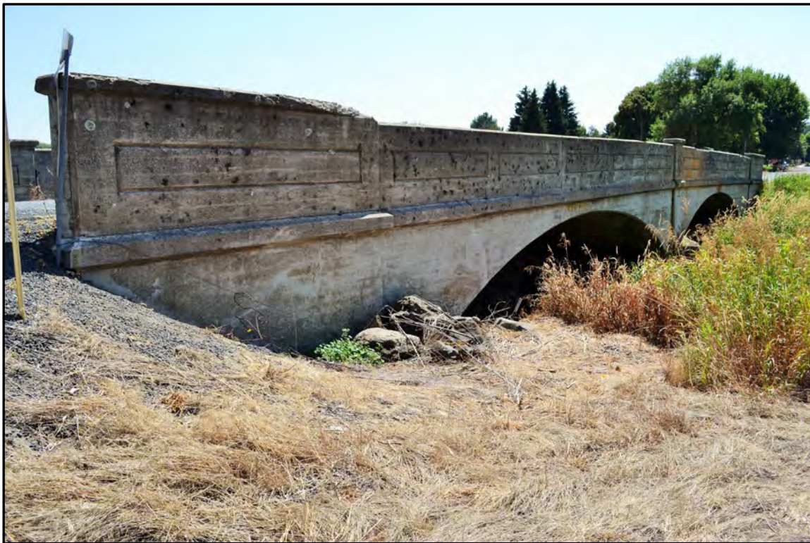
Figure A-44. Colton Bridge No. 37 (Field Number WCLB-7), west side; view to the southeast.
