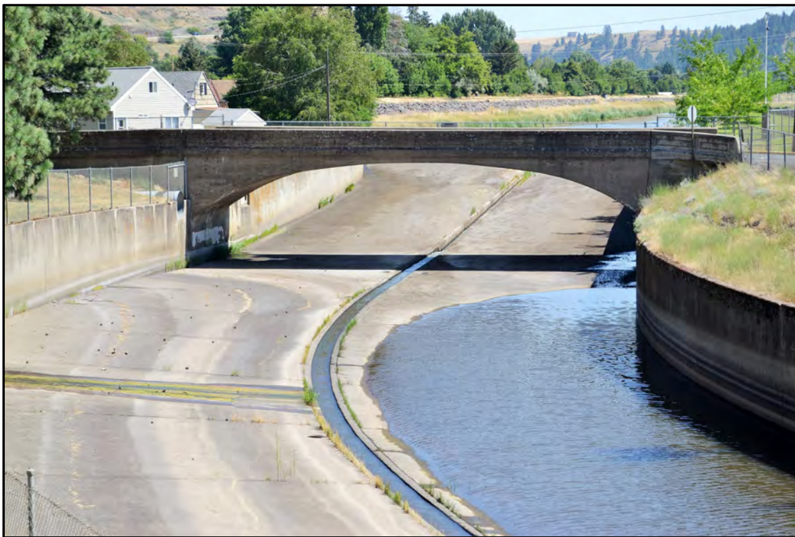
Figure A-56. Mill Dam Bridge (Field Number WCLB-9), west side; view to the northeast. The bridge's north arch is buried under the fill to the left of the channelized river.
