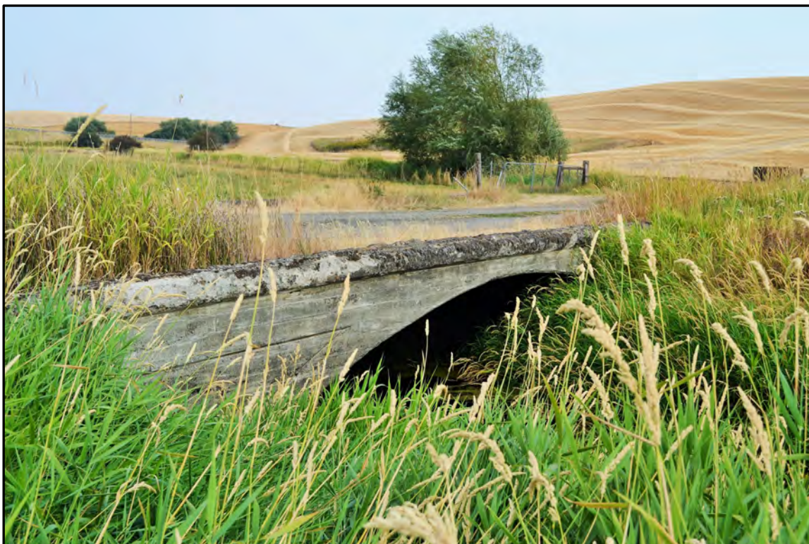
Figure A-111. Kelley Bridge (Field Number WCLB-16), west side; view to the southeast.
