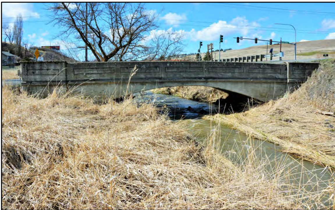
Figure A-77. Wood Bridge (Field Number WCLB-11), east side; view to the northwest (photograph courtesy of Whitman County Public Works).
