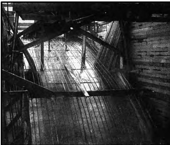
Figure 19. Steel reinforcing rods in place, Maumee Bridge, Waterville, Ohio, before 1909 (National Bridge Company 1908:138).
