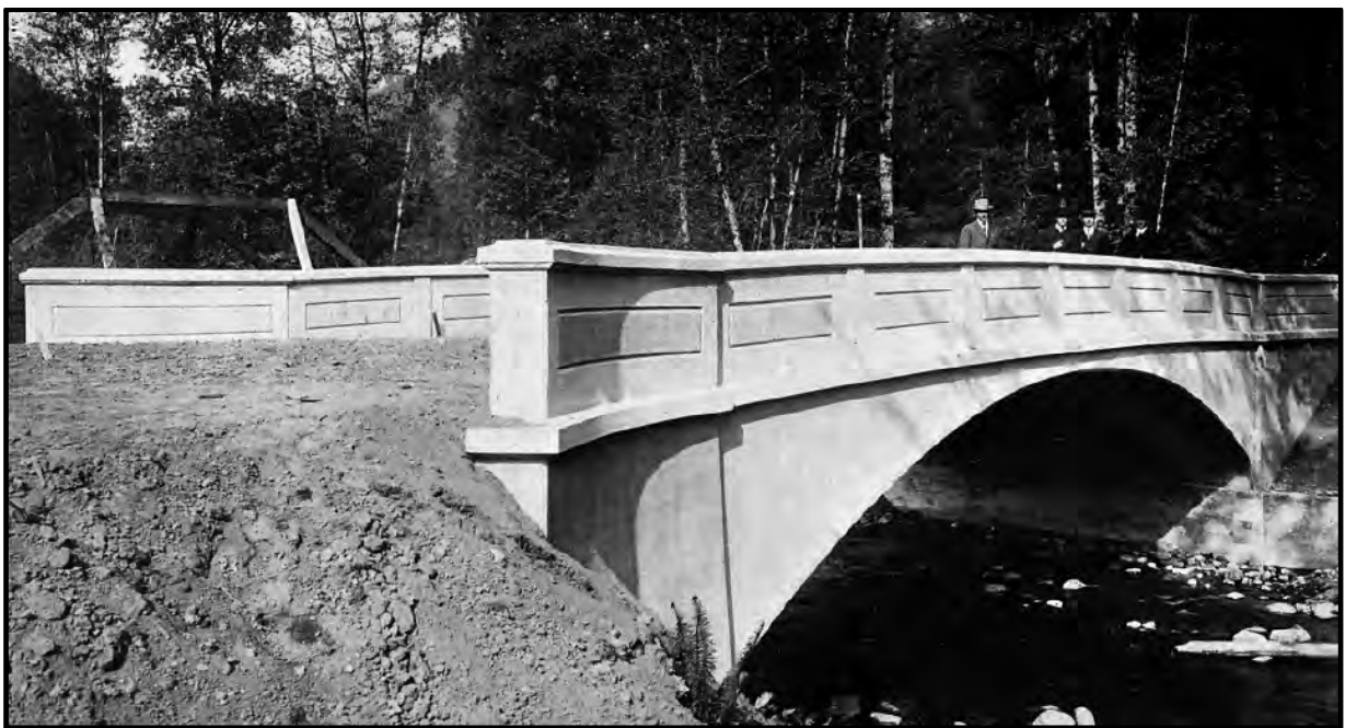
Figure 13. Raging River Bridge, King County, Washington, built 1916 (Luten 1917:38)
