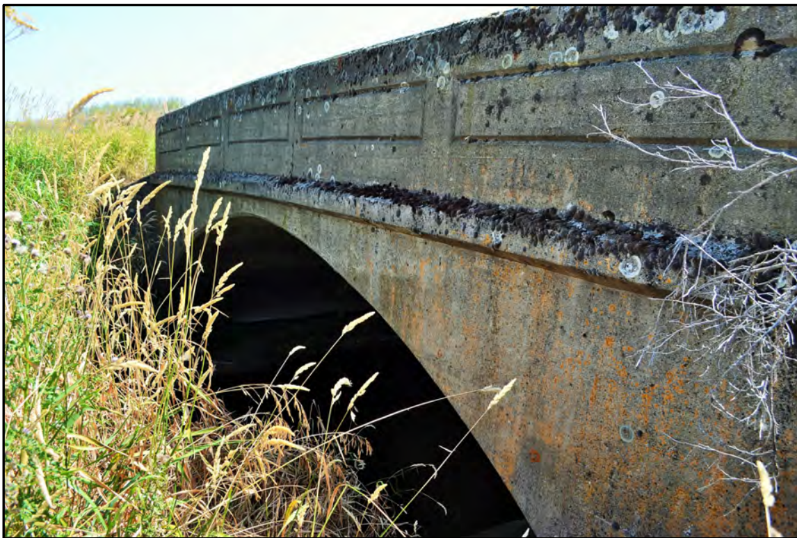
Figure A-85. Devine Bridge (Field Number WCLB-12), west side; view to the northeast.
