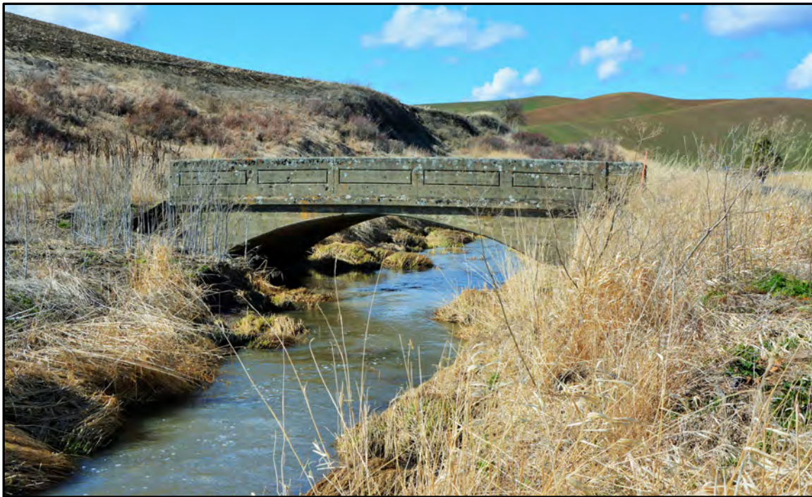
Figure A-84. Devine Bridge (Field Number WCLB-12), east side; view to the northwest (photograph courtesy of Whitman County Public Works).
