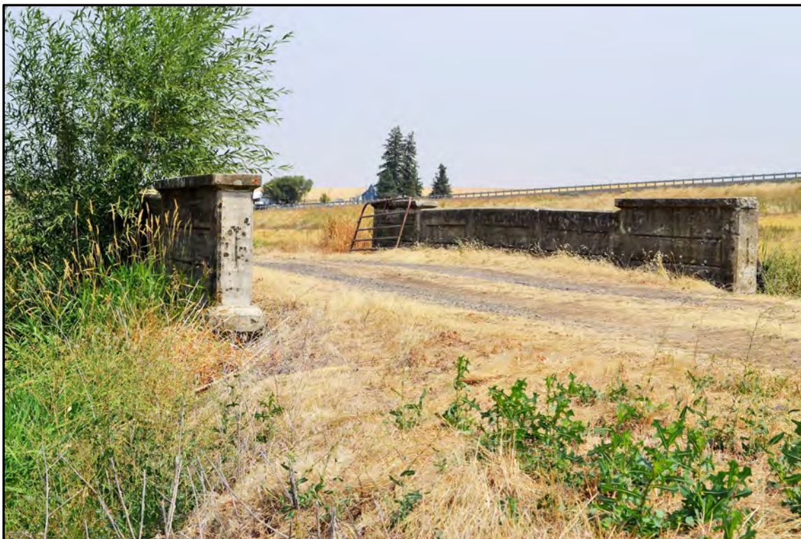
Figure A-91. Bridge No. 317 (Field Number WCLB-13), south approach and west side; view to the northeast.
