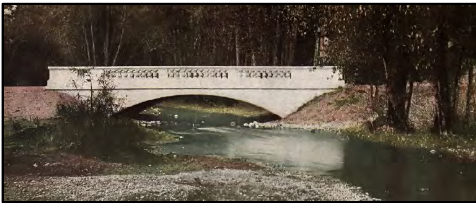
Figure 15. Clover Creek Bridge, Pierce County, Washington, built 1914 (Luten 1917:36)
