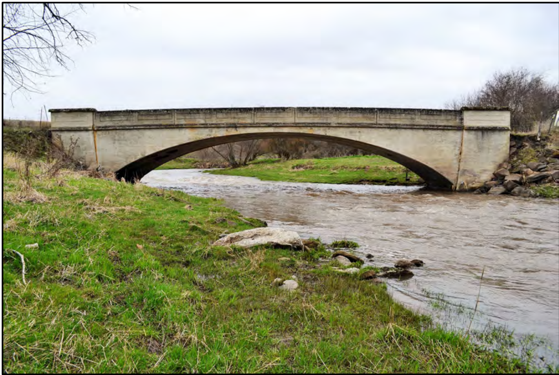
Figure A-2. Kenova Bridge (Field Number WCLB-1), west side; view to the southeast.
