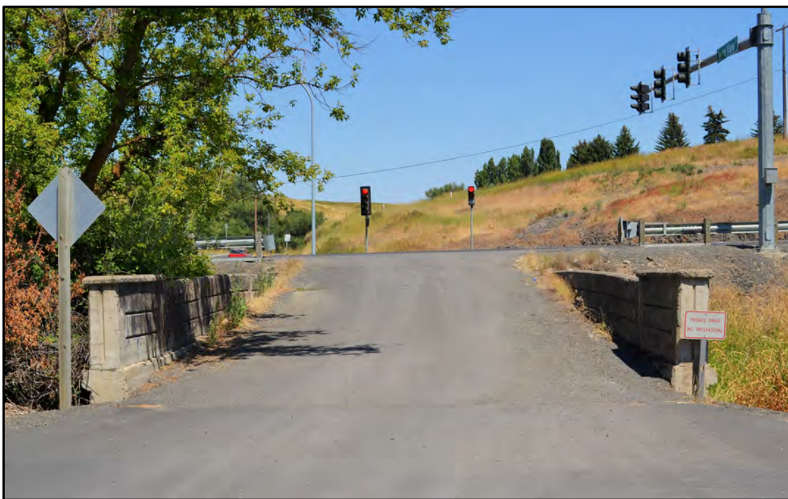
Figure A-79. Wood Bridge (Field Number WCLB-11), south approach; view to the north. The road conveyed by the bridge has been built up to the level of State Route 270, which is visible in the background.
