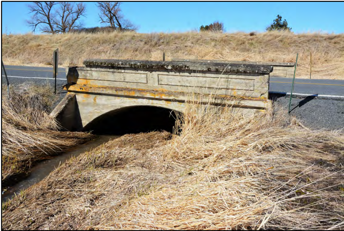
Figure A-38. Colton Bridge (Field Number WCLB-6), east side; view to the northwest (photograph courtesy of Whitman County Public Works).
