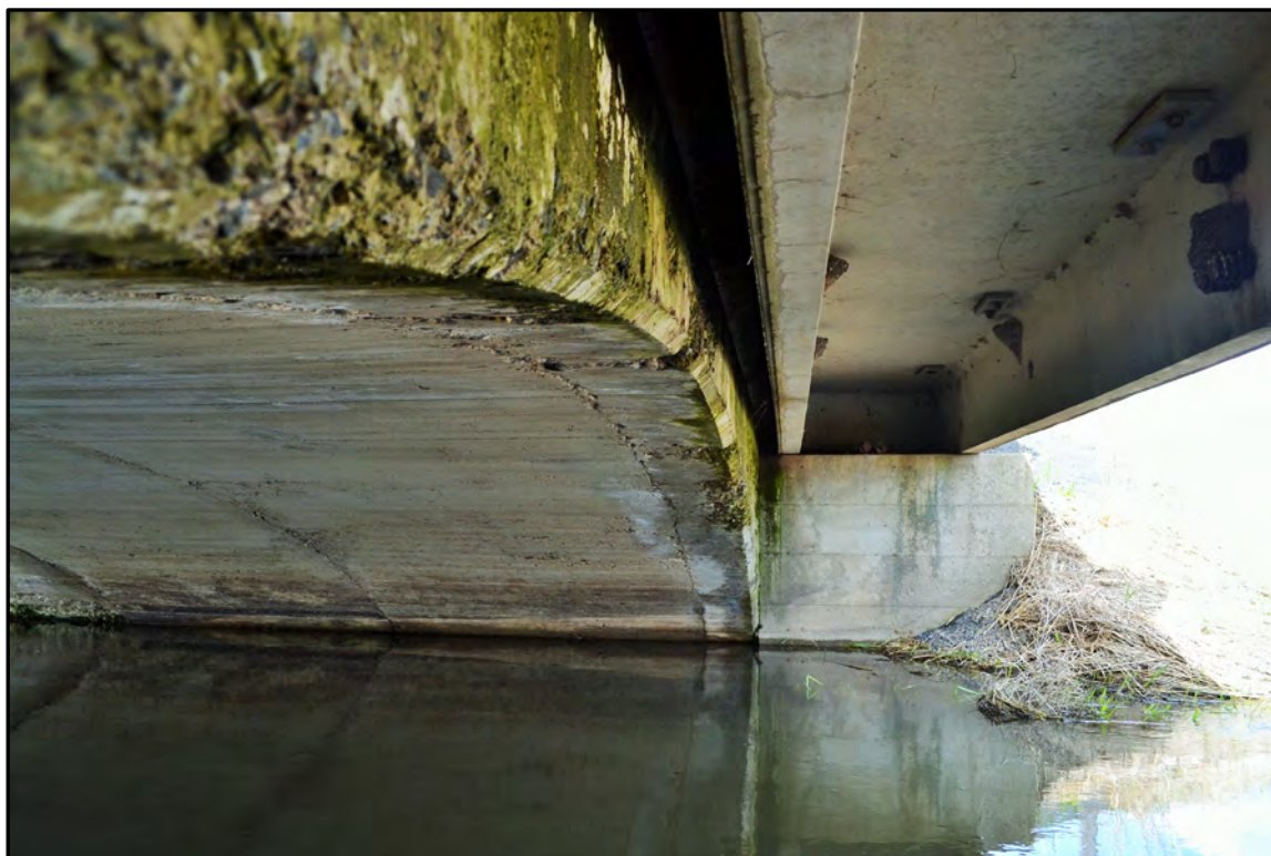
Figure A-25. Morley Bridge (Field Number WCLB-4), north end of arch barrel with girder added to widen road; view to the northwest.
