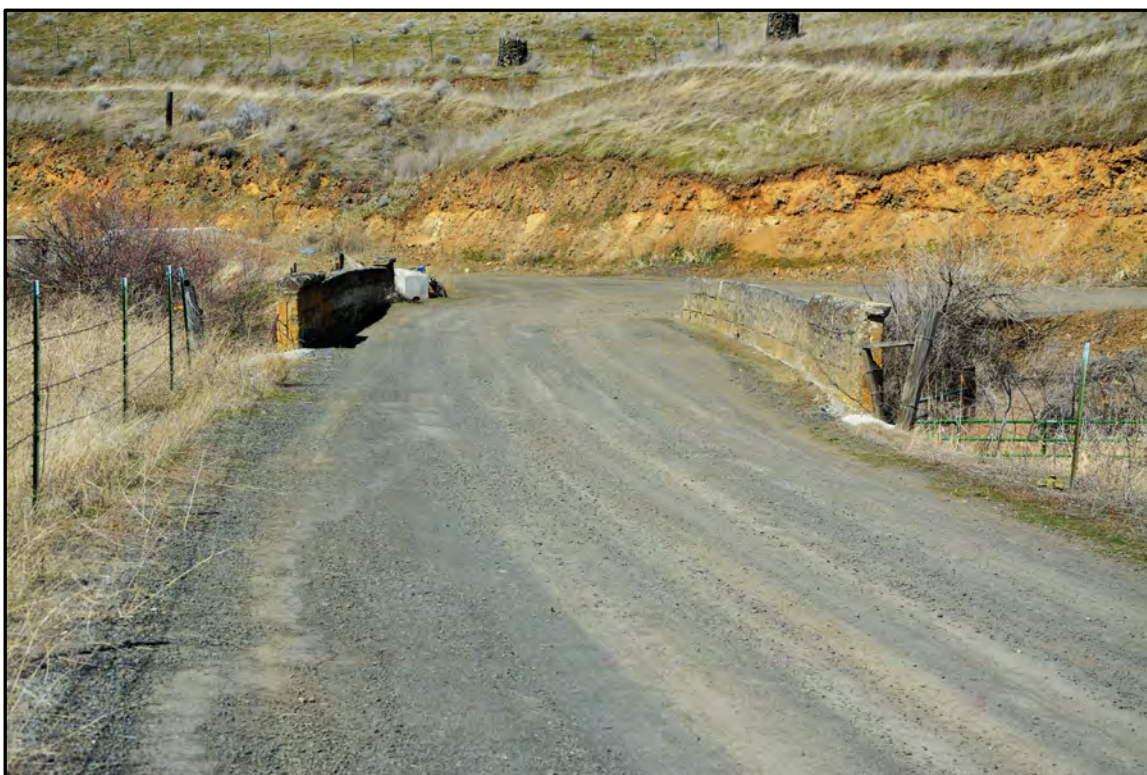
Figure A-104. Rhodes Bridge (Field Number WCLB-15), south approach; view to the northwest (photograph courtesy of Whitman County Public Works).
