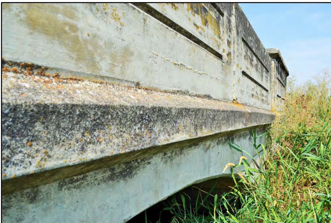
Figure A-92. Bridge No. 317 (Field Number WCLB-13), detail of east side; view to the north.
