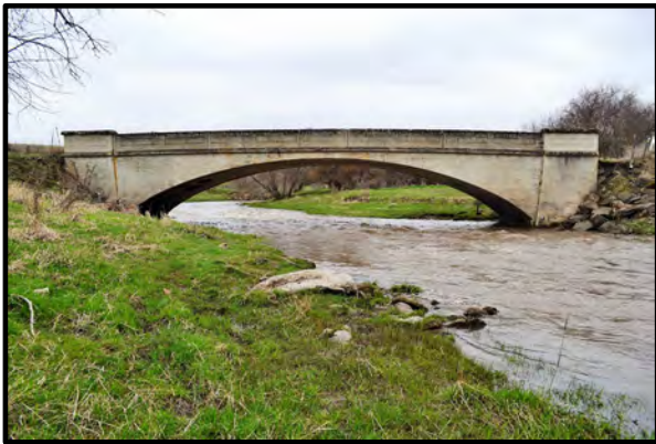
Figure 23. Kenova Bridge (Field Number WCLB-1), west side; view to the southeast.
