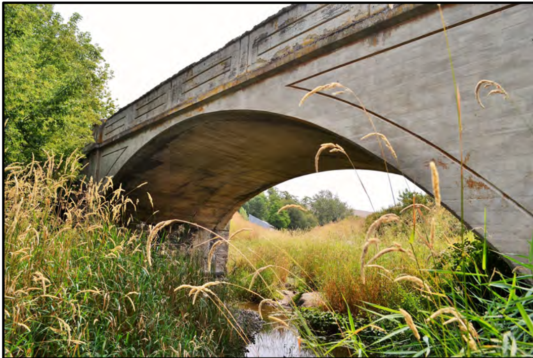
Figure 2. Sanders Bridge (Field Number WCLB-17), north side of west arch; view to the southeast.
