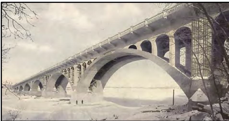
Figure 16. Saskatchewan River Bridge, Saskatoon, Saskatchewan, built 1915 (Luten 1917:4).
