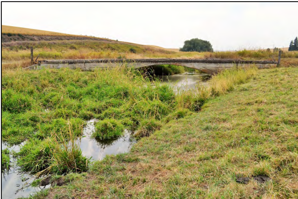
Figure A-109. Kelley Bridge (Field Number WCLB-16), east side; view to the southwest.
