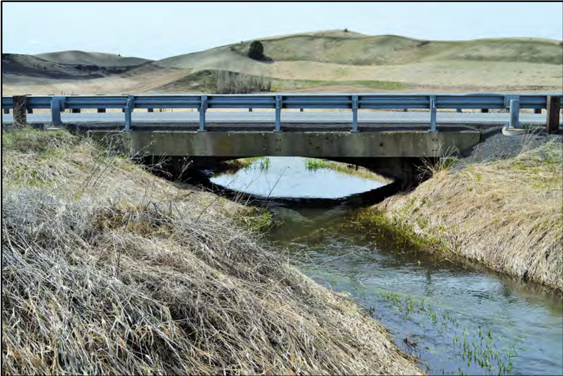
Figure A-23. Morley Bridge (Field Number WCLB-4), east side; view to the west. Note girder added to widen the road.
