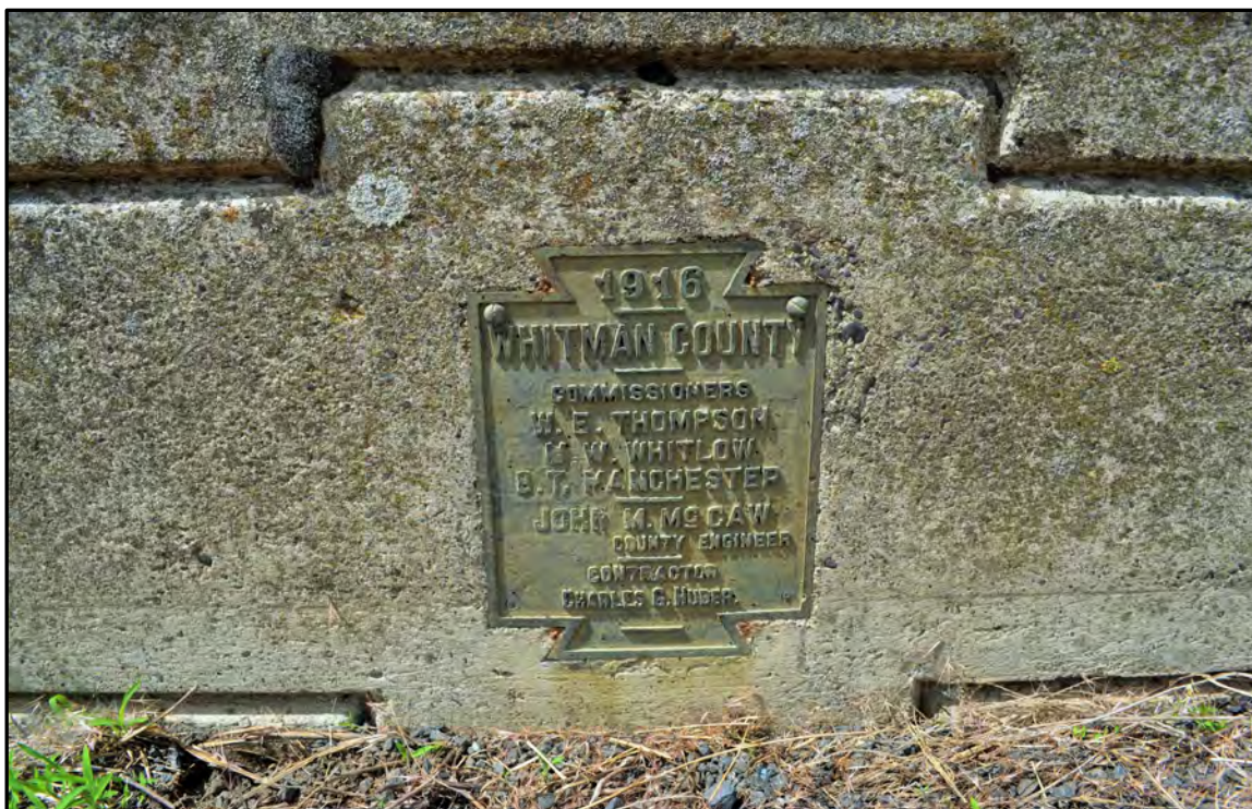
Figure A-11. McLeod Bridge (Field Number WCLB-2), plaque on inner west parapet; view to the southwest.
