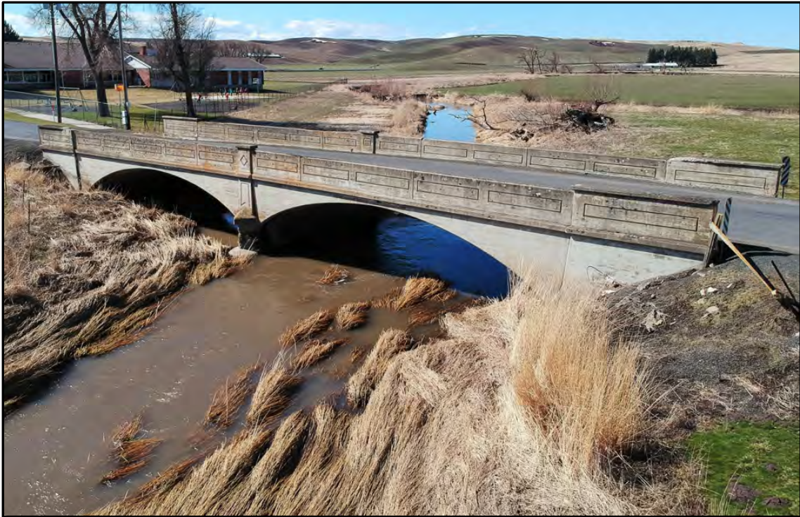
Figure A-43. Colton Bridge No. 37 (Field Number WCLB-7), east side; view to the southwest (photograph courtesy of Whitman County Public Works).
