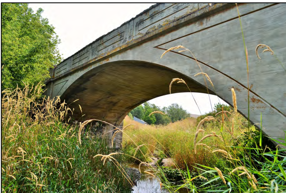
Figure A-118. Sanders Bridge (Field Number WCLB-17), north side of west arch; view to the southeast.
