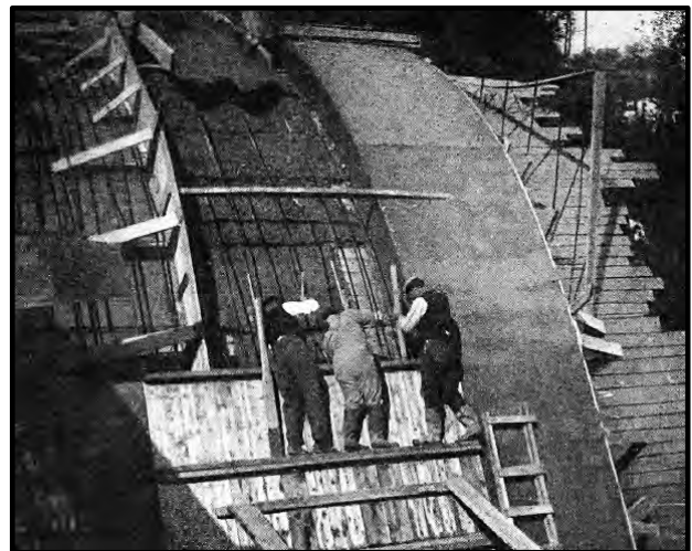
Figure 20. Pouring arch ring concrete, unidentified bridge, Plymouth, Massachusetts, before 1909 (National Bridge Company 1908:139).
