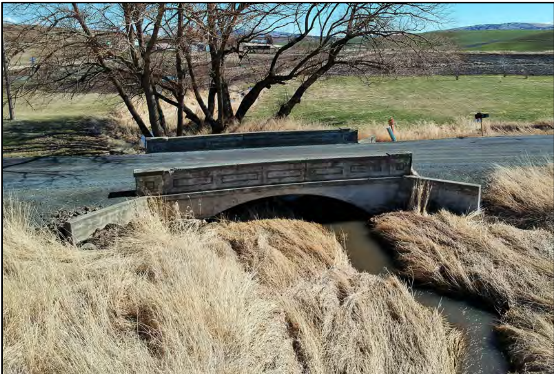
Figure A-29. Staley Bridge (Field Number WCLB-5), west side; view to the southeast (photograph courtesy of Whitman County Public Works).
