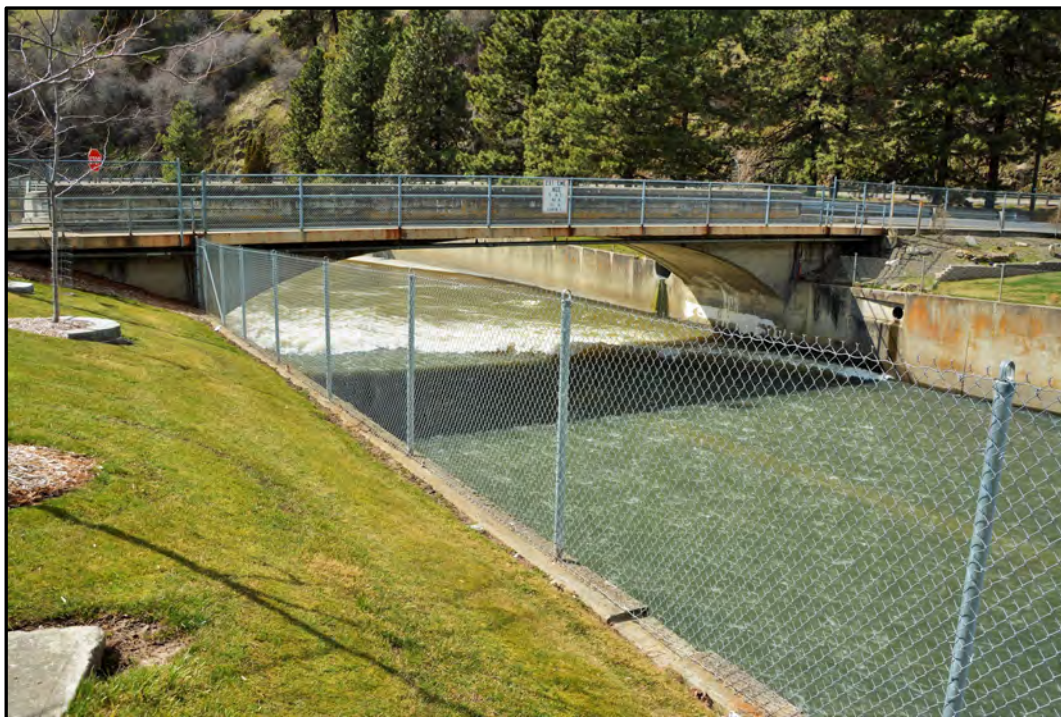
Figure A-57. Mill Dam Bridge (Field Number WCLB-9), east side; view to the southwest. The bridge's north arch is buried under the fill to the right of the channelized river (photograph courtesy of Whitman County Public Works).
