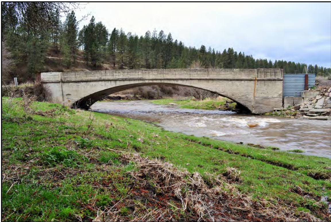
Figure A-3. Kenova Bridge (Field Number WCLB-1), east side; view to the northwest.
