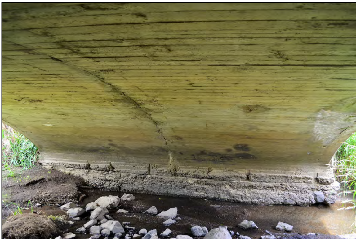
Figure A-18. Seltice Bridge (Field Number WCLB-3), south part of arch barrel; view to the southeast.
