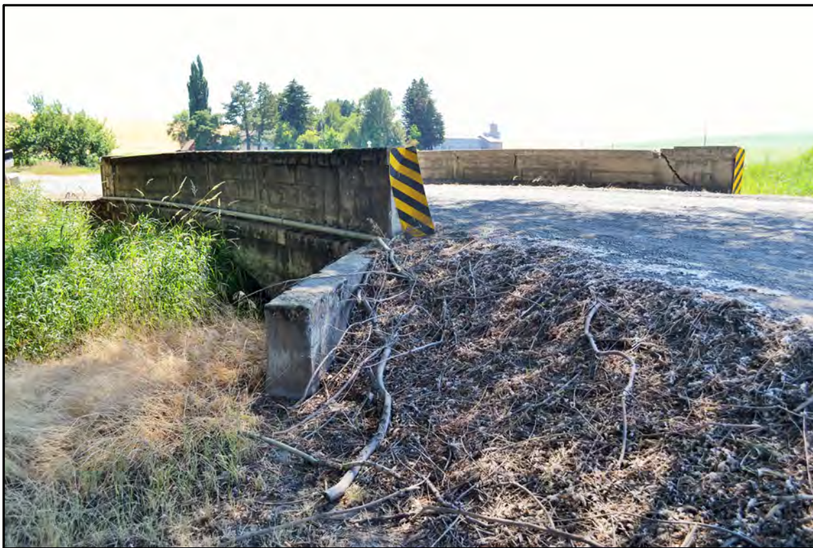
Figure A-30. Staley Bridge (Field Number WCLB-5), east side; view to the southwest.
