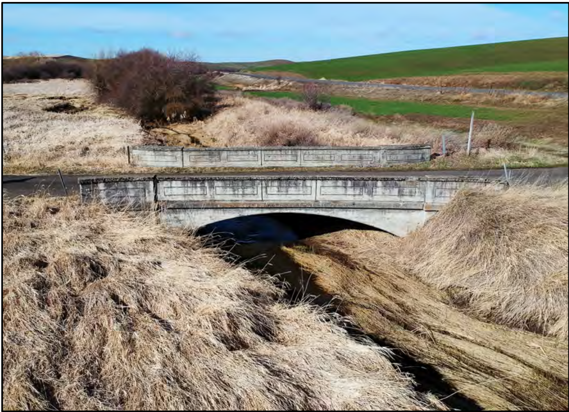
Figure A-16. Seltice Bridge (Field Number WCLB-3), east side; view to the west (photograph courtesy of Whitman County Public Works).
