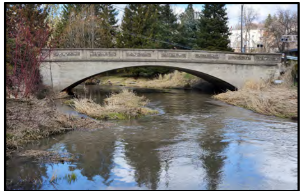
Figure 26. Spring St. Bridge (Field Number WCLB-10), south side; view to NE (Whitman Co. photo).
