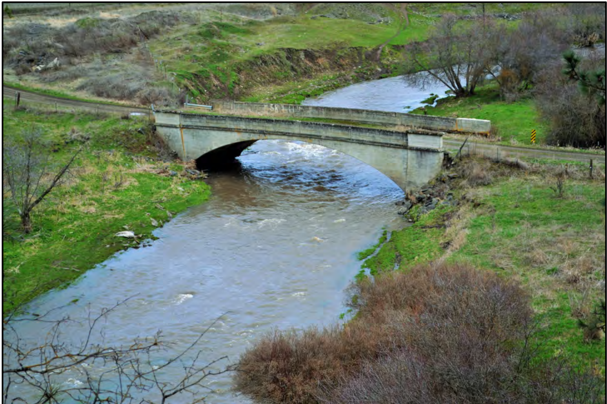
Figure A-1. Kenova Bridge (Field Number WCLB-1), west side as viewed from Hole-in-the-Ground Road; view to the northeast.
