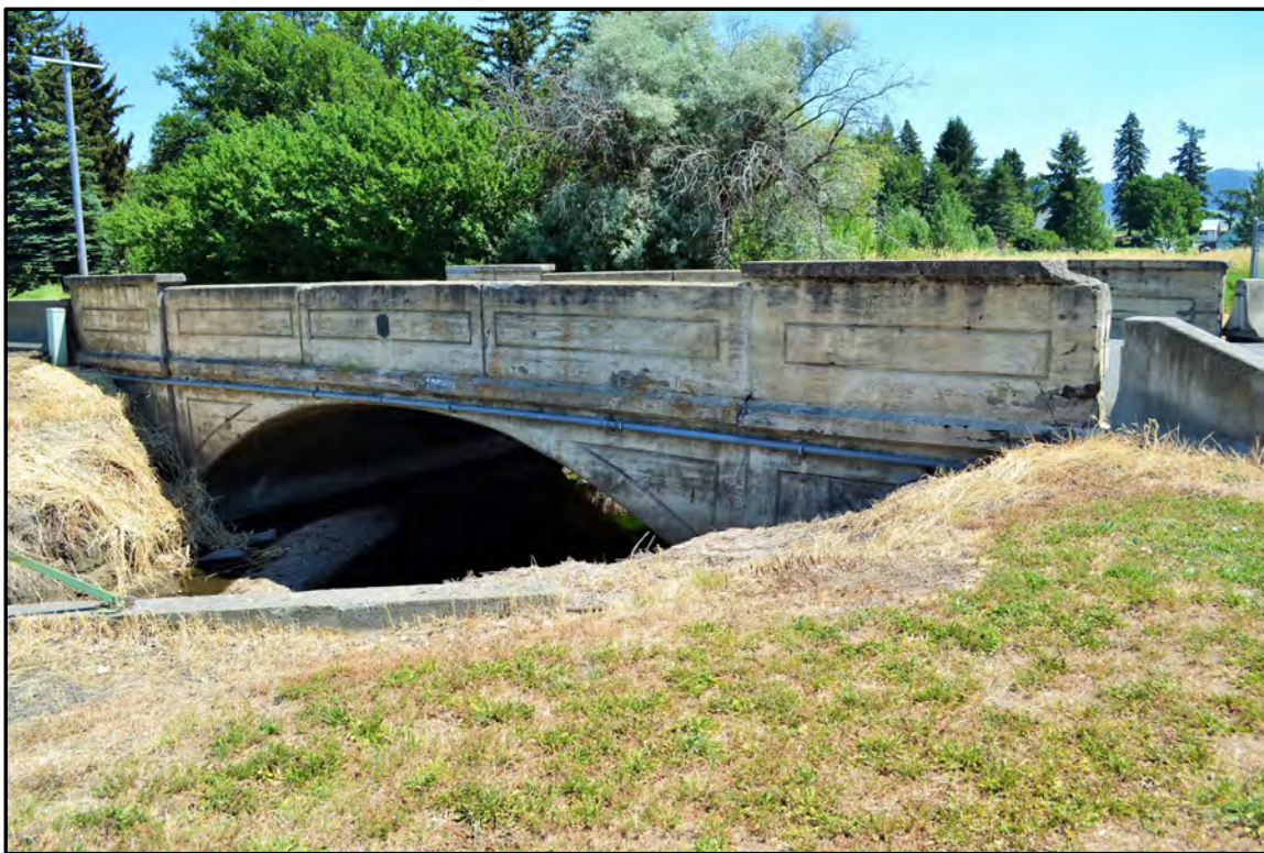
Figure A-51. First Street Bridge (Field Number WCLB-8), west side; view to the northeast.
