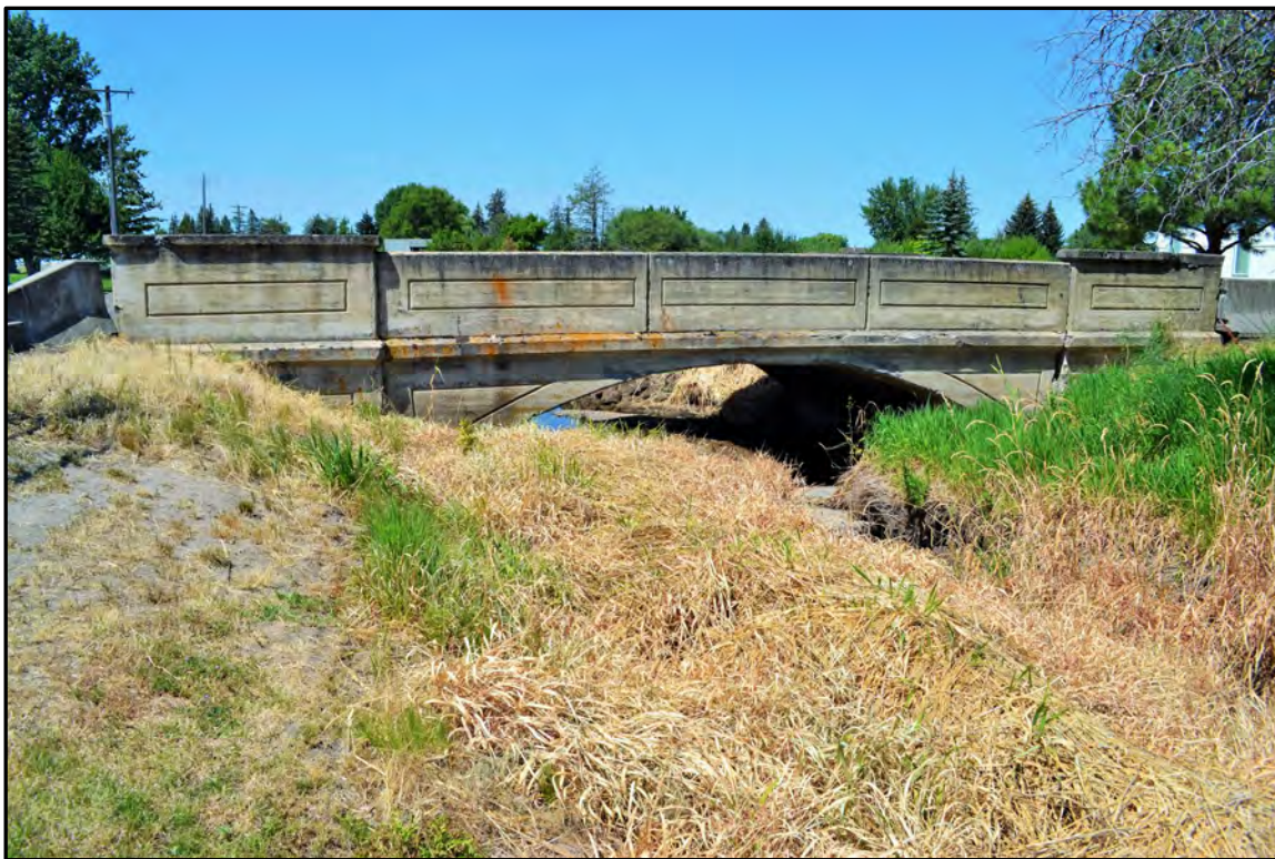
Figure A-50. First Street Bridge (Field Number WCLB-8), east side; view to the northwest.
