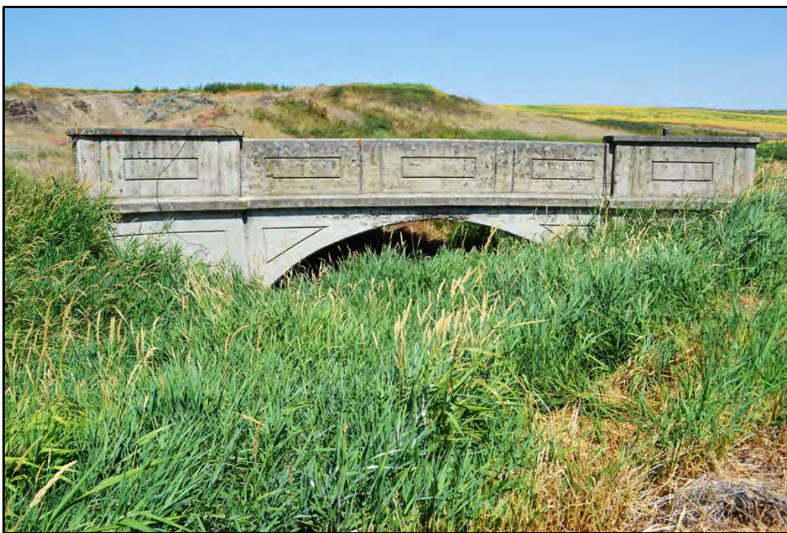
Figure A-97. Bridge No. 318 (Field Number WCLB-14), west side; view to the northeast.
