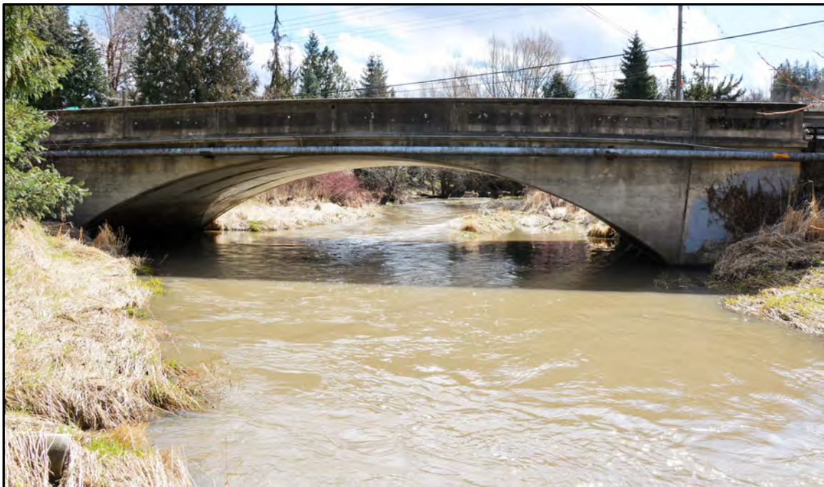
Figure A-71. Spring Street Bridge (Field Number WCLB-10), north side; view to the southeast (photograph courtesy of Whitman County Public Works).
