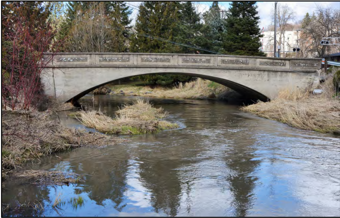
Figure A-70. Spring Street Bridge (Field Number WCLB-10), south side; view to the northeast (photograph courtesy of Whitman County Public Works).
