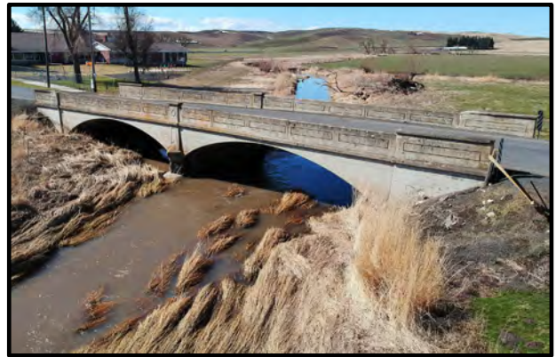
Figure 24. Colton Bridge (Field Number WCLB-7), east side; view to southwest (Whitman Co. photo).
