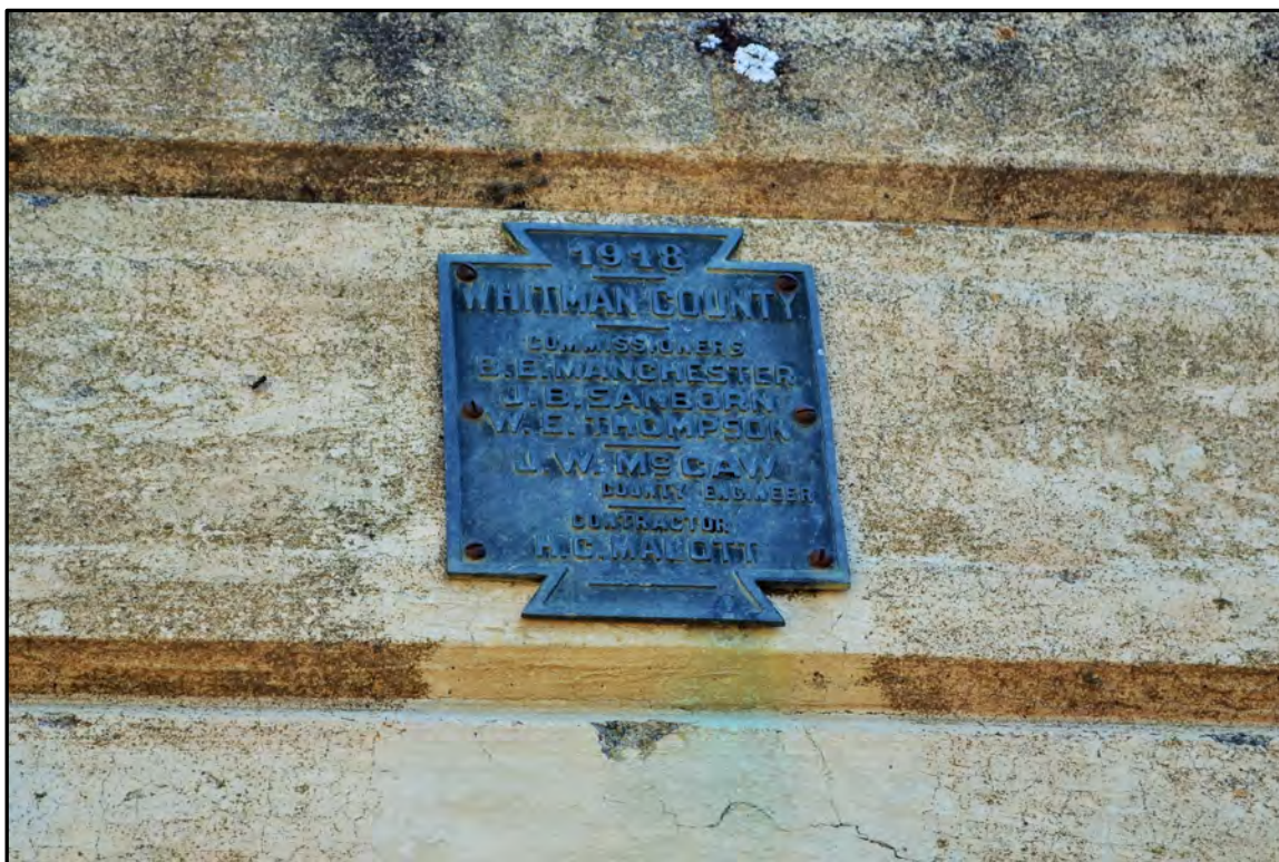
Figure A-52. First Street Bridge (Field Number WCLB-8), plaque on exterior side of west parapet; view to the east.
