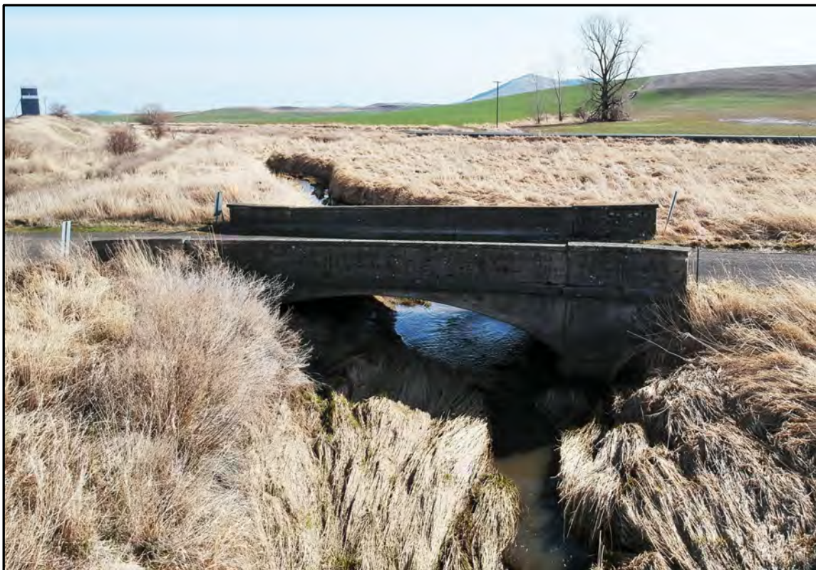
Figure A-17. Seltice Bridge (Field Number WCLB-3), west side; view to the east (photograph courtesy of Whitman County Public Works).
